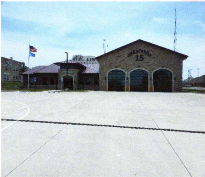
Rolling Meadows Station 15 at 3201 Algonquin Rd
