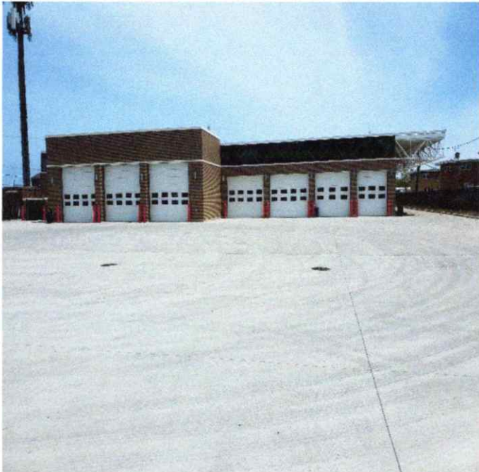
Mount Prospect Station 13 at 111 East Rand Rd
